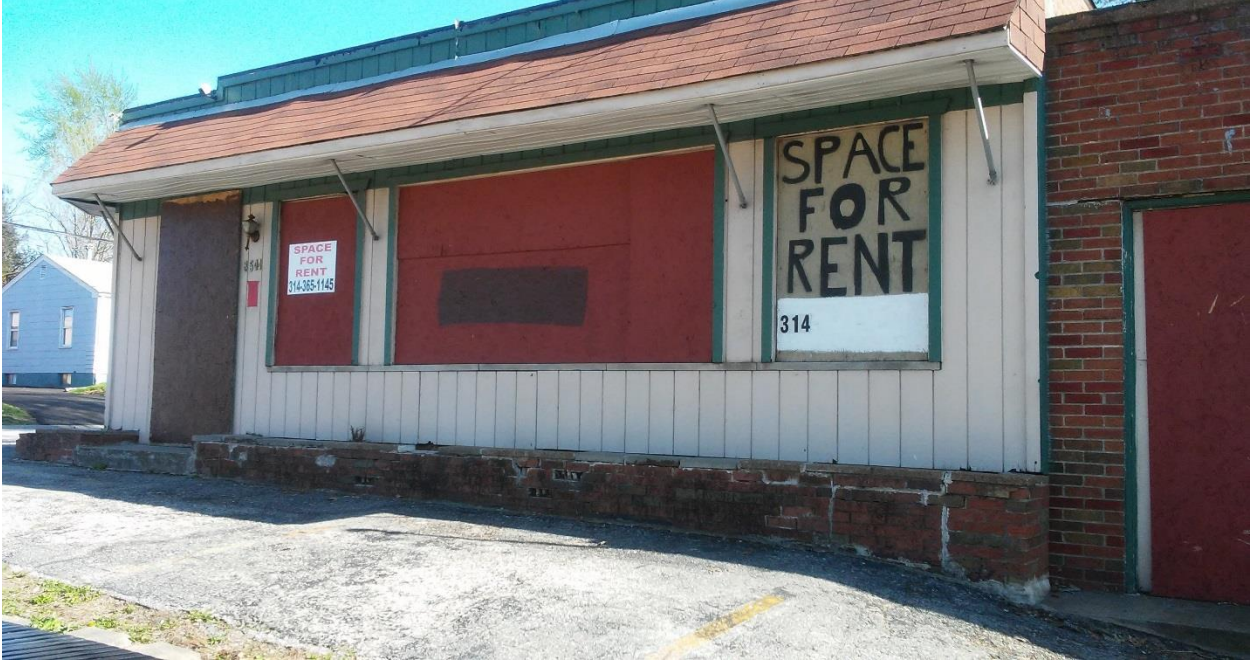
FRONT OF BUILDING (ENTRANCE DOOR AND EMERGENCY EXIT DOOR)
