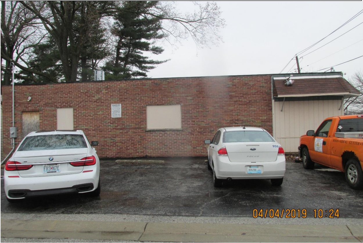
SIDE OF BUILDING: (PARKING LOT ON GARFIELD)
